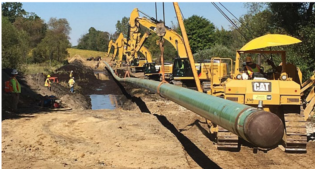
Figure 17: Illustrative pipeline installation 41
