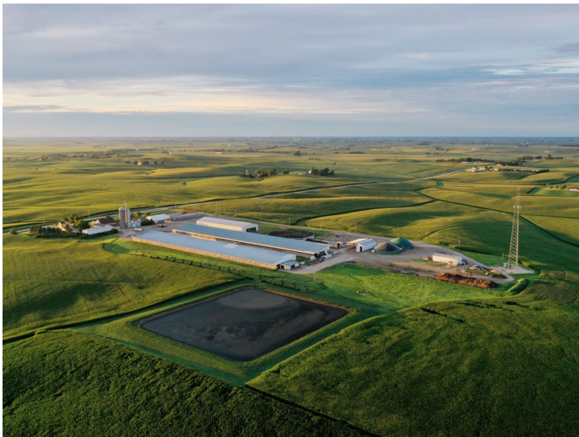
Figure 2. Large Midwest anaerobic digestion facility.
