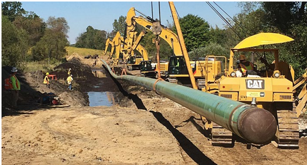
Figure 17: Illustrative pipeline installation 41
