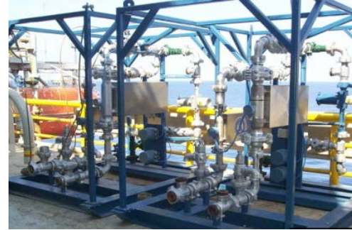
Slip Stream at Wellhead (with BP & Schlumberger)
